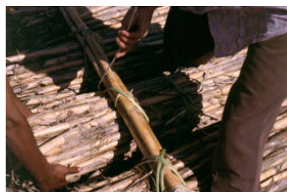
Fig. 6. Construction of a cane pontoon raft on the Moroccan coast of Gibraltar Strait, 7 October 1999.
